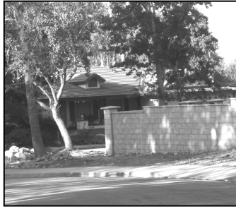
Split-faced decorative block wall with decorative cap along a street facing side property line
