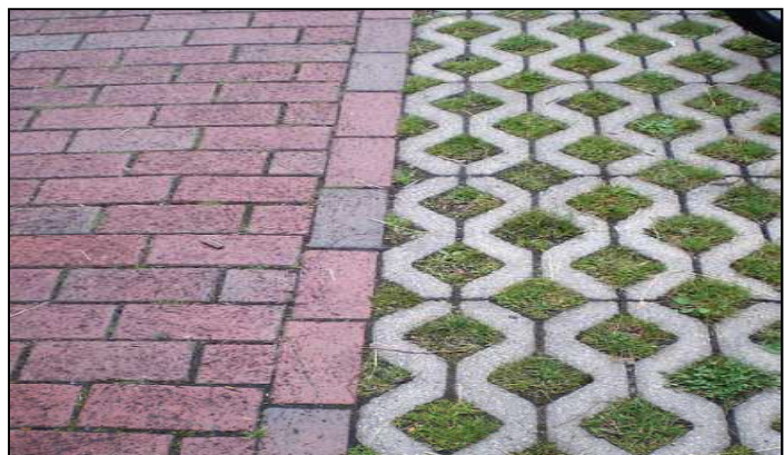
Pervious Paving
