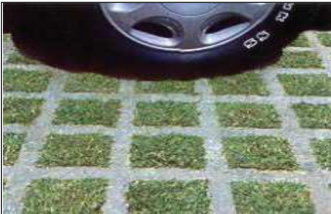
Pervious Paving
