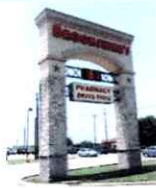
Sign support wrapped in masonry
