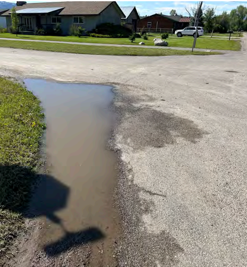
FIRST & FREEMONT AVENUE
