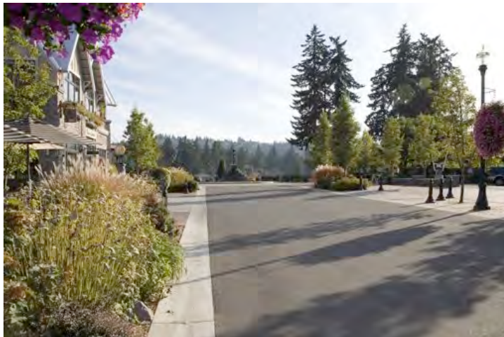
Example of Drainage Ribbon and Potential Stormwater Planter/Snow Storage Area on Side Streets
