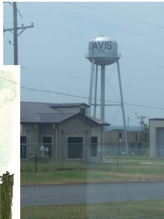
Water Plant Tower
